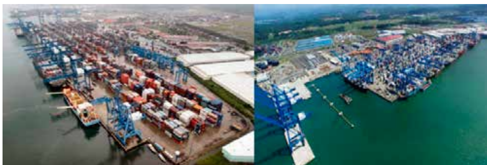
Figura 139 Manzanillo International Terminal
