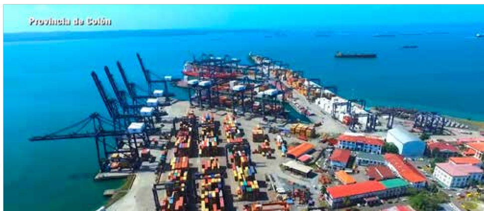
Figura 127 Vista Panama Ports Company (PPC)
